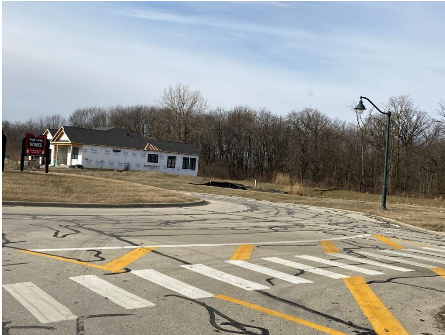
Photo 3: View of villa under construction on Lot 50.
